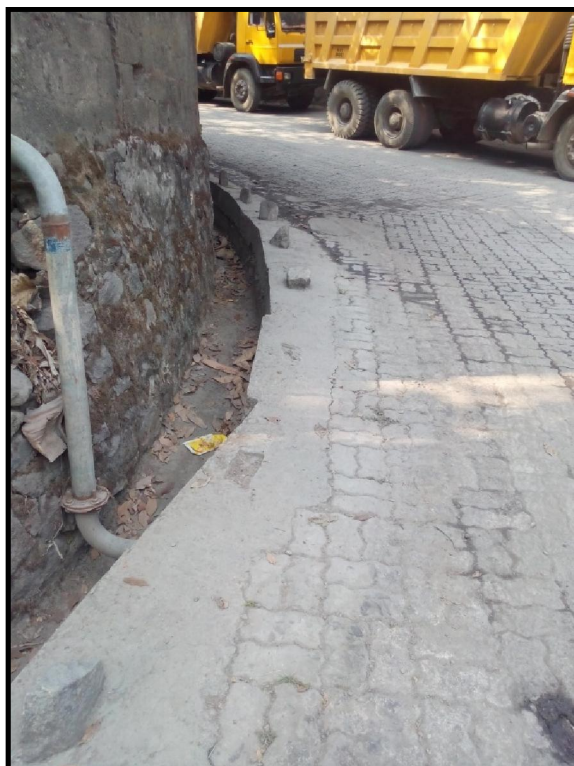
Photographs showing garland drains to channelize storm water
