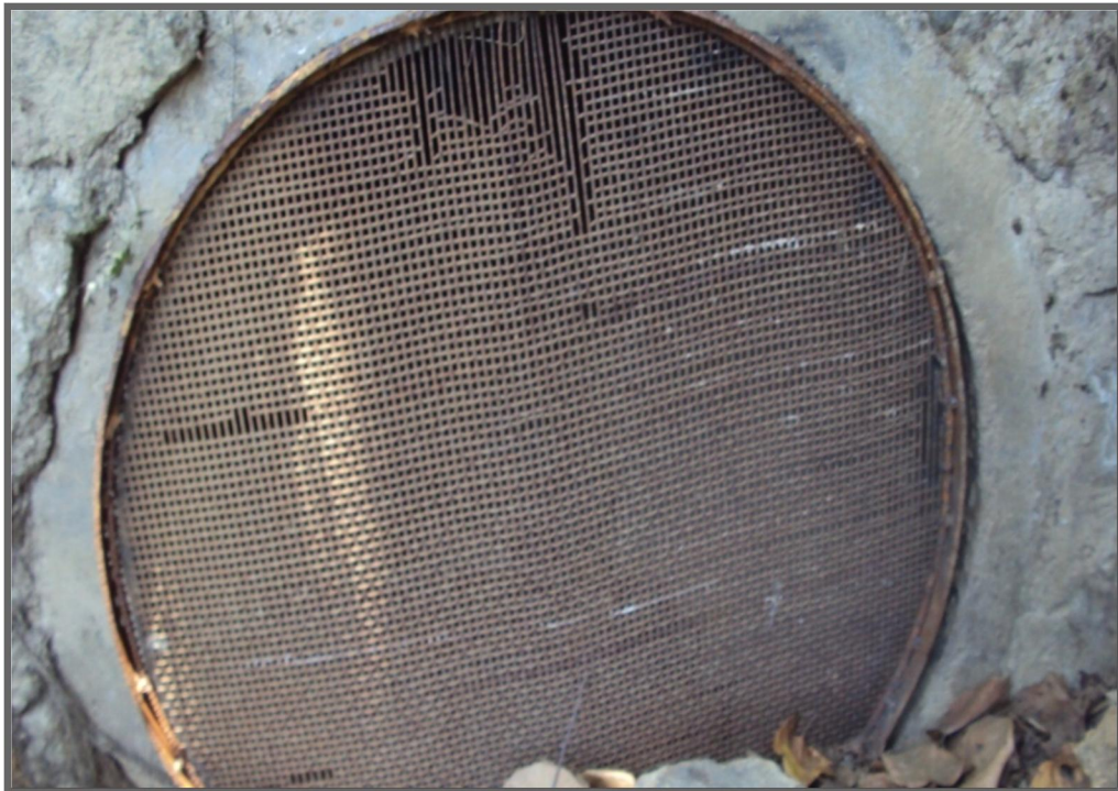
Photographs showing the storm water storage pit and debris/silt traps to prevent entry of quarry waste to the main streams.
